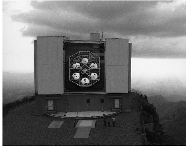
**Fig. 3** The original Multiple Mirror Telescope on Mount Hopkins, Arizona, consisting of six 1.8-m mirrors in a common mount and with a common focus. Photo: Smithsonian Institution Archives.
